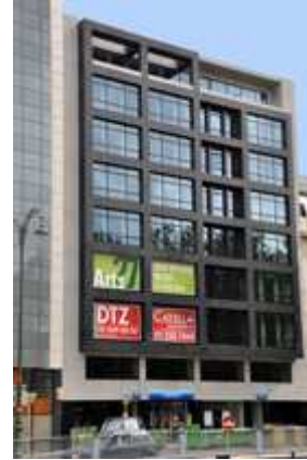
Exhibit 16 Arts 27 (after redevelopment), Brussels
